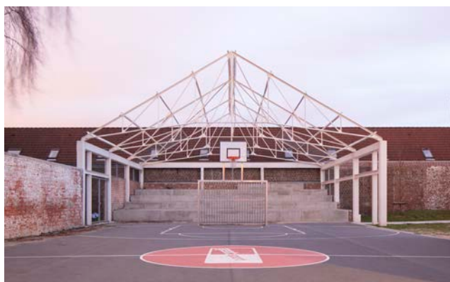
Ref. Multifunctionele verharde ruimte: parking, basketbalveld, tribune,... - De Pore, Gent
