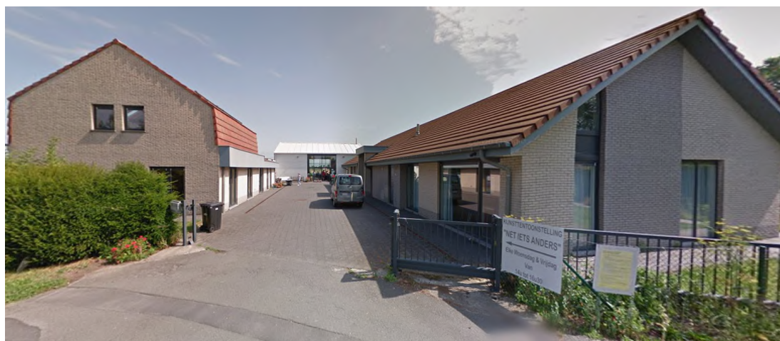
Figuur 4 – Site De Bollaard (bron: Google Streetview)
